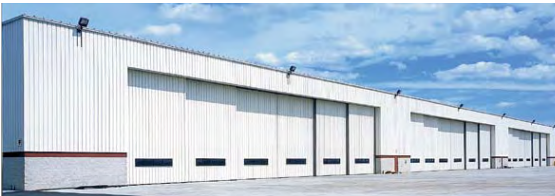
The giant building’s 500-foot clearspan took custom engineering and a reverse-frame design.
